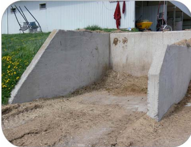
Figure 6. Storage in the side of a hill makes it easy to dump wheelbarrows. Install safety stops at the top edge.
