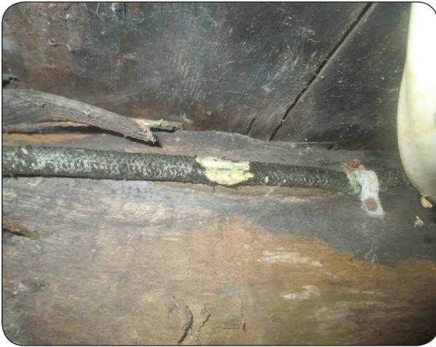
**Figure 5.** Rodent damage on electrical cable.
