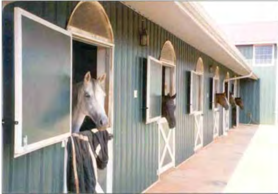
Fig. 7. Horses in this barn have egress through doors to the inside aisleway as well as to the outside. Dutch doors or paddocks off of each stall are highly recommended to allow responders access to animals even after smoke and fire are present. Photo courtesy of Dr. Tomas Gimenez.
