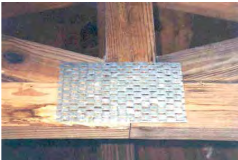
Fig. 11. Joist connectors or gusset plates. Photo courtesy of Tomas Gimenez.
