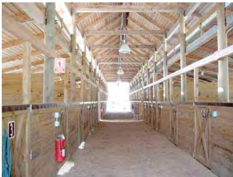
Fig. 9. The interior hallway of a well-constructed horse barn with post and beam. Note the safety features: all electrical in conduit, fire extinguishers, multiple exits, emergency lighting, ventilation, and easily opened latches. Photo courtesy of Tomas Gimenez.
