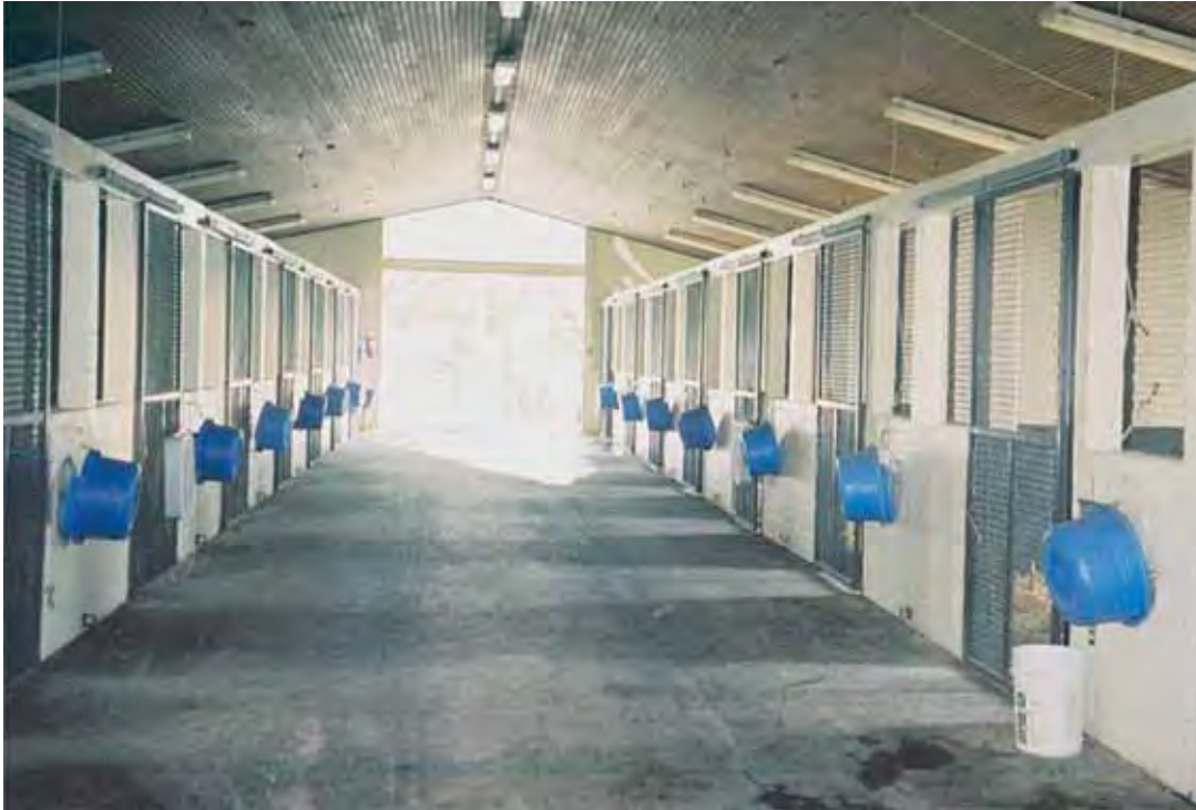
Fig. 10. The interior hallway of another well-constructed barn showing metal-rafter construction, hoses, doors to both the interior and exterior wall, and wide aiseways. Photo courtesy of Tomas Gimenez.
